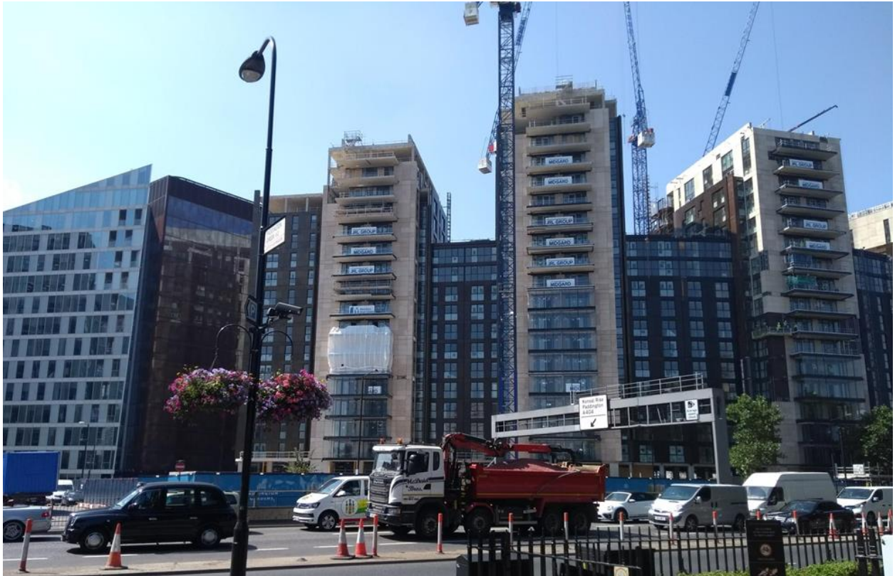
View of site from north side of the Westway (A40) – site in foreground in front of residential blocks under construction.
